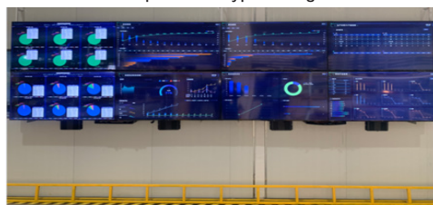
Dali Base Data Monitoring Screen
